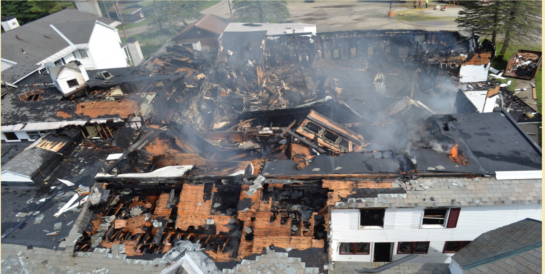
Rutland Town plywood manufacturing plant destroyed by fire. This fire resulted in millions of dollars in property damage and loss of many jobs
