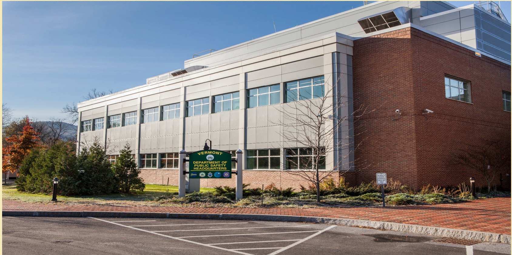
External view of the Vermont Forensic Laboratory
