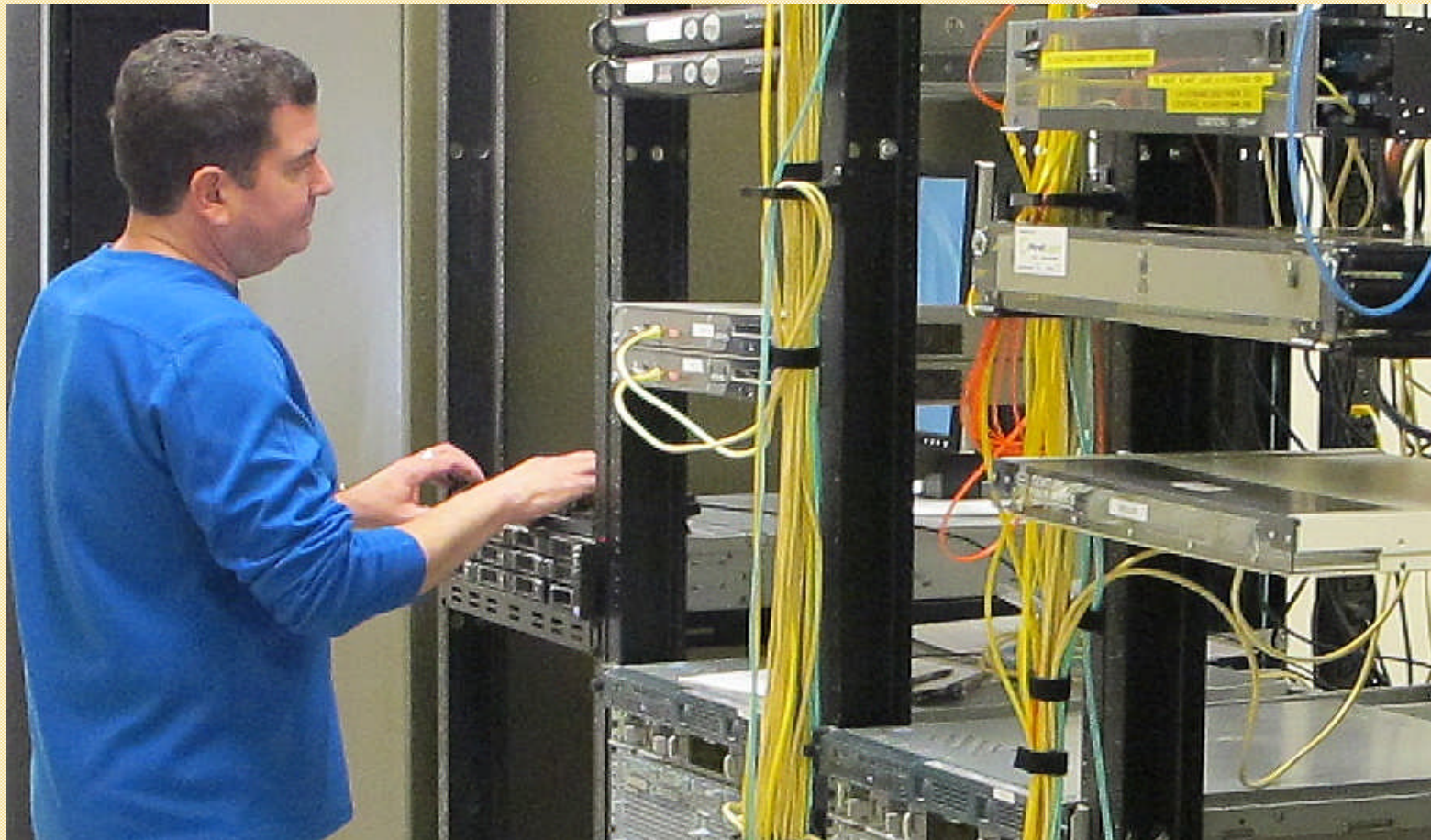
Server Room- Virtual and Physical server environment housed at DPS
